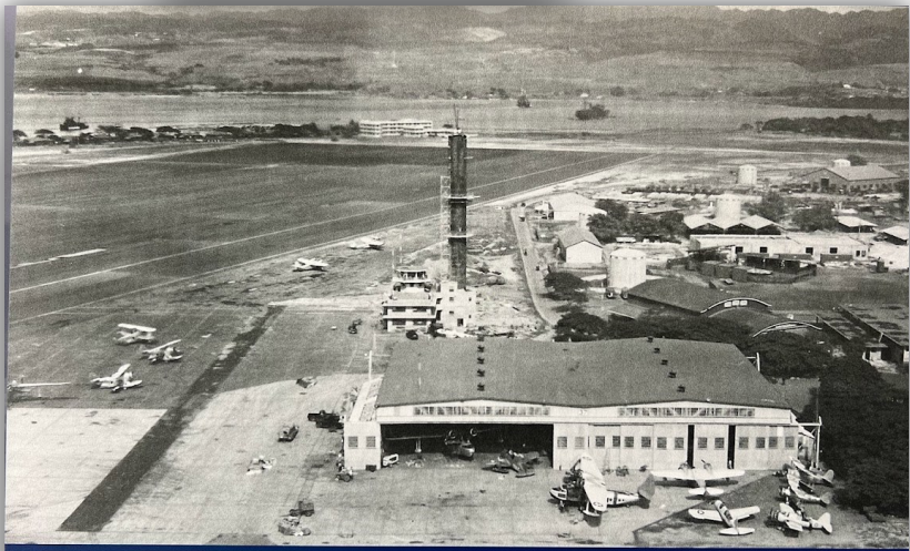
Building S84 on December 8, 1941. You can see that the upper control tower was not yet built. Construction of the 156-foot control tower began in early 1941. At the time of the Japanese attack on Pearl Harbor, the tower structure was about 80% complete and without the aircraft control tower on the top. Courtesy of the National Archives (80-G-32482)
