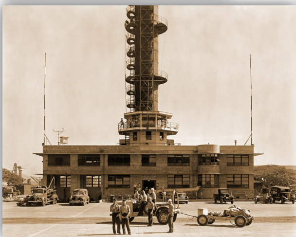
Building S84 on December 8, 1941. You can see that the upper control tower was not yet built. Construction of the 156-foot control tower began in early 1941. At the time of the Japanese attack on Pearl Harbor, the tower structure was about 80% complete and without the aircraft control tower on the top. Courtesy of the National Archives (80-G-32482)
